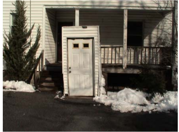
A pretty grand entry to get to the unfinished basement.
