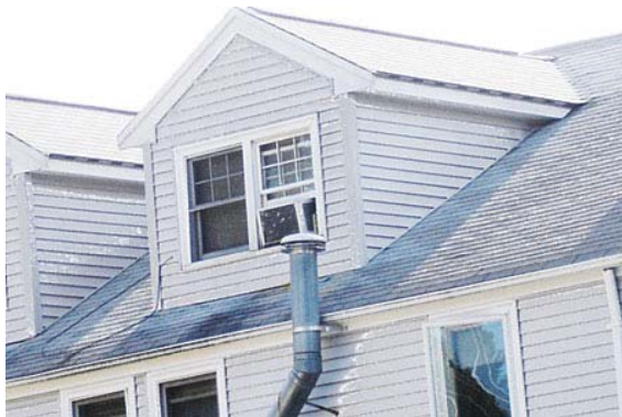
Exhaust could send Carbon Monoxide into room with A/C from Bob Mulloy East Bridgewater, MA
